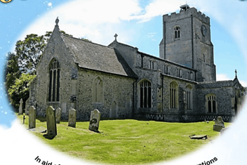
In aid of Dullingham Church path and clock renovations
